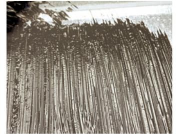
If utilizing a roller, use a medium to thick knap roller, typically ¾" or taller.
