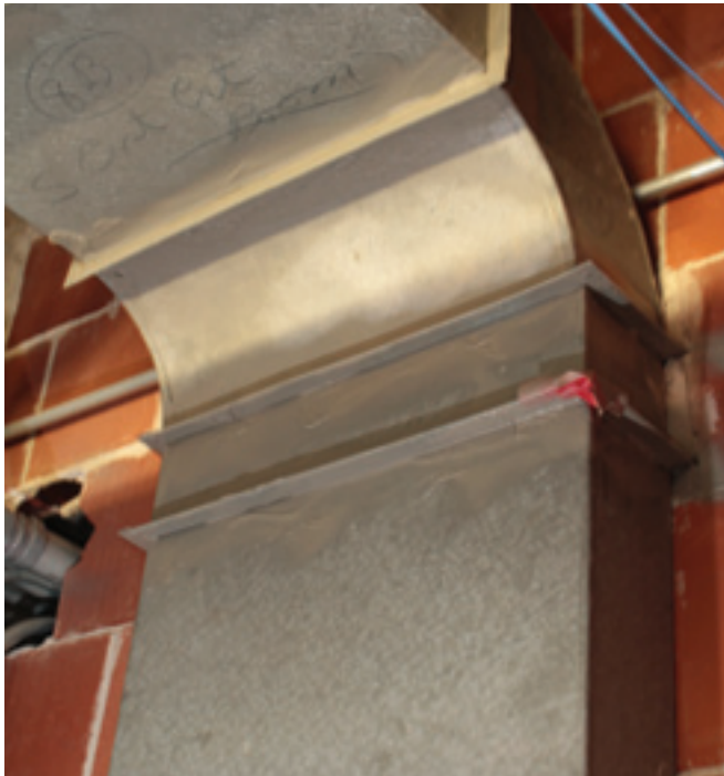
The Oklahoma courthouse's ductwork was sealed with Spray-Seal from Hardcast.
